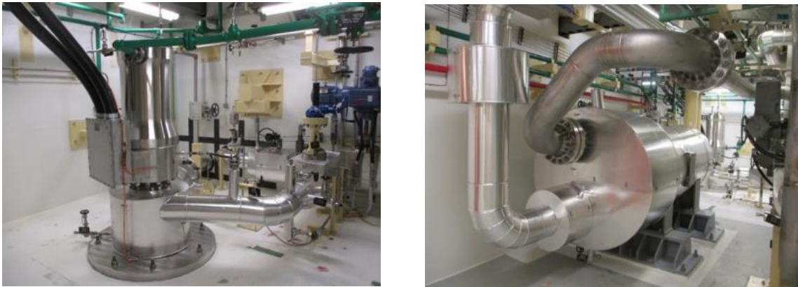
Figure 29: External Connection Point for ARHR System Cooling Water
