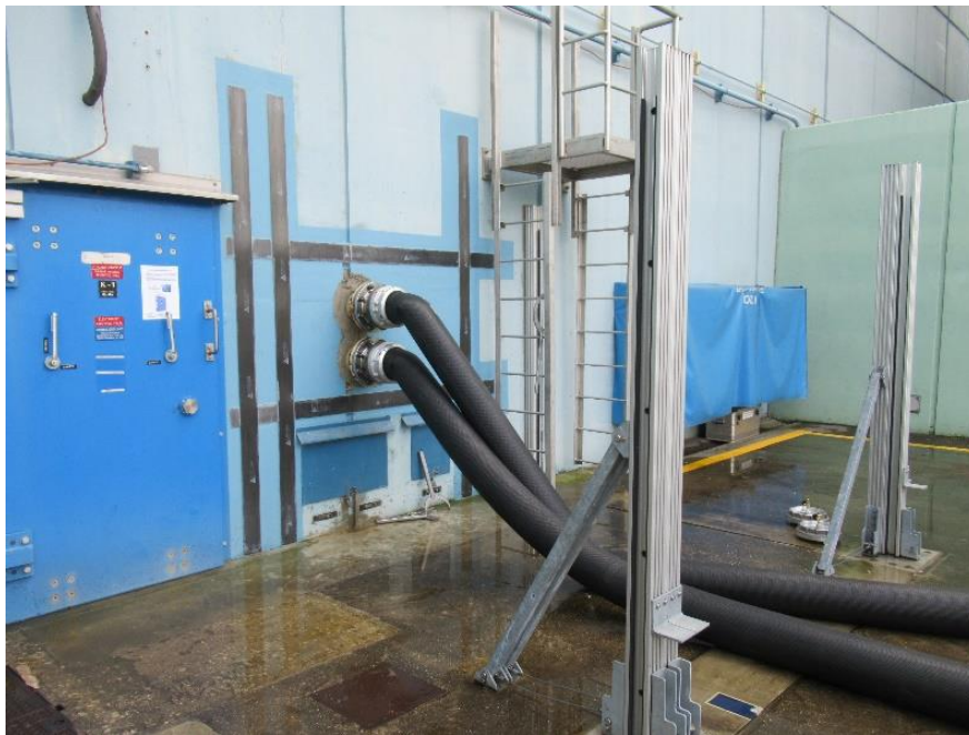
Figure 29: External Connection Point for ARHR System Cooling Water
