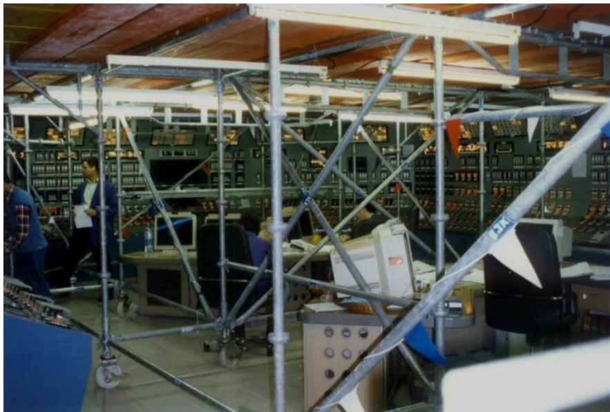
Figure 32: Replacement of MCR Ceiling with Fire Resistant Material
