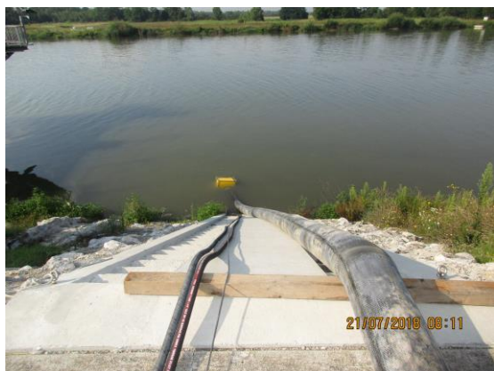
Figure 34: Pumping Station with Floating Pump
