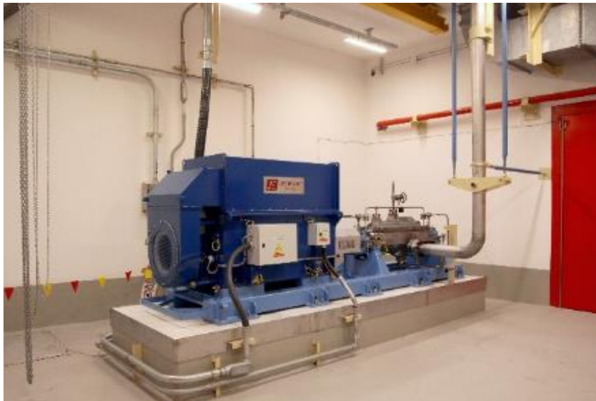
Figure 27: Alternative Auxiliary Feedwater Pump (AAF)
