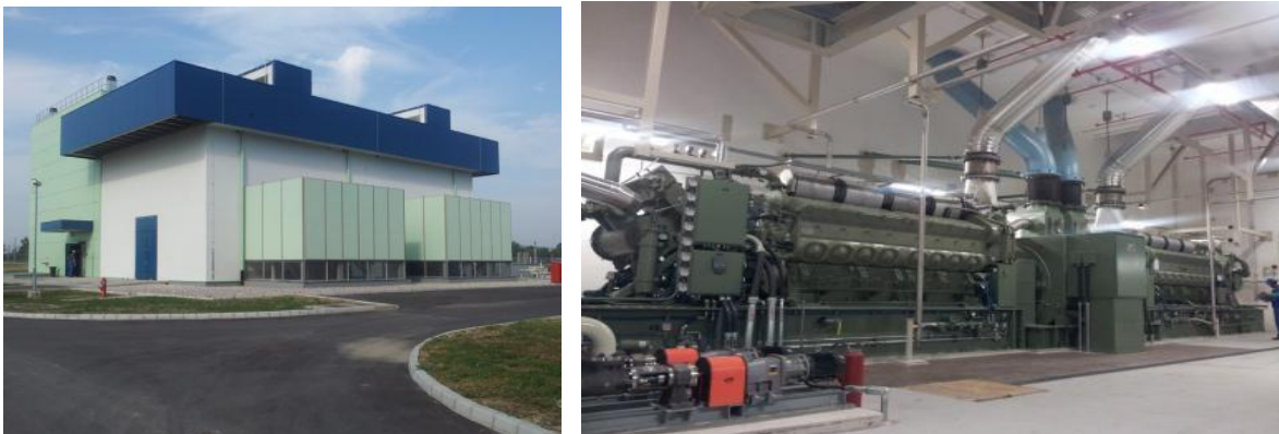
Figure 24: Bunkered Building and Emergency Diesel Generator 3
