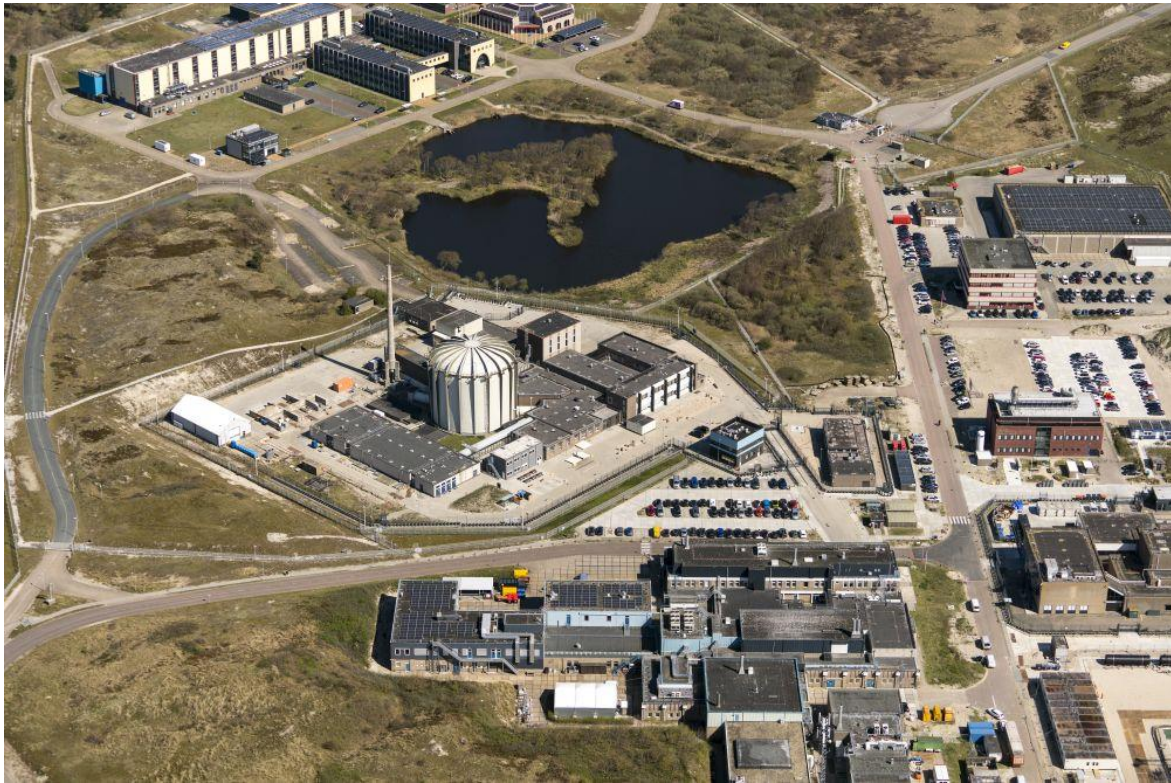
Figure 1.3 Aerial view of RR HFR and its surroundings
