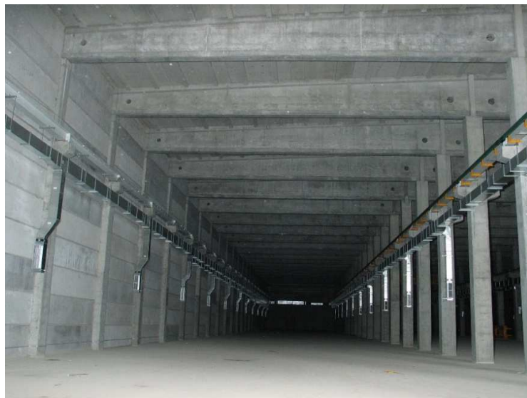
Figure 2.2.5-2. Partial inside view of the building 158/2
