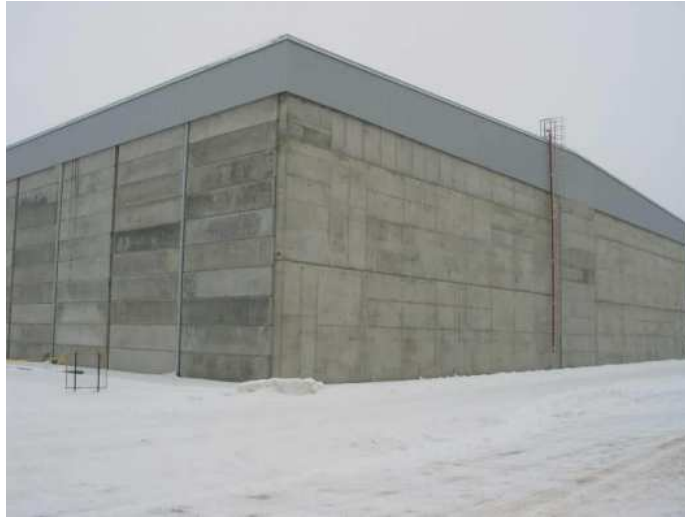
Figure 2.2.5-1. Partial view of building 158/2.
