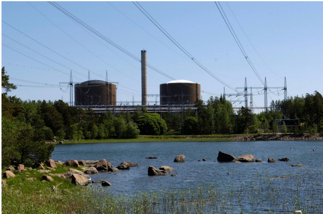
Figure 1. Loviisa nuclear power plant (image source: Fortum)
