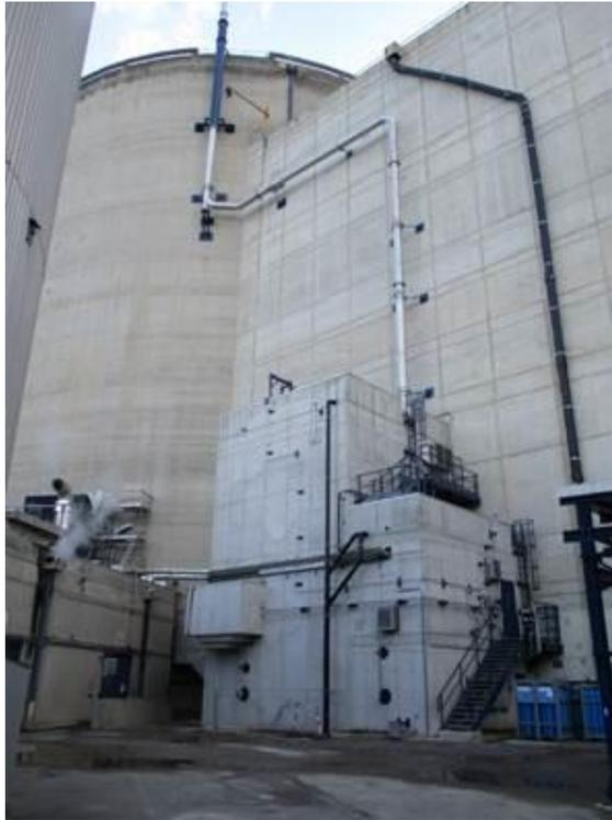
Figure 4 : Filtered containment venting systems of Tihange 3
