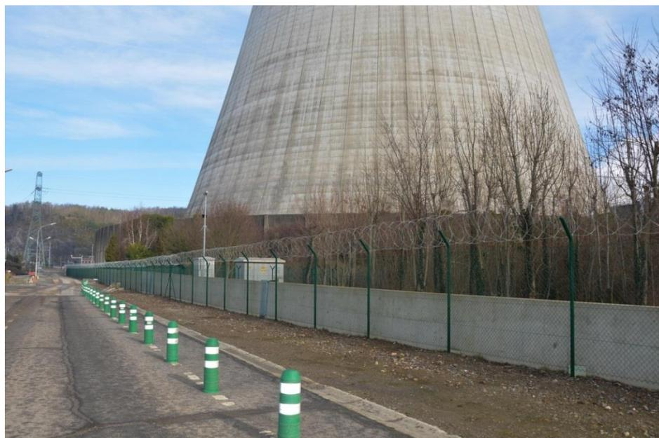
Figure 2: Peripheral protection of the site of Tihange against beyond-design flooding realized in 2015
