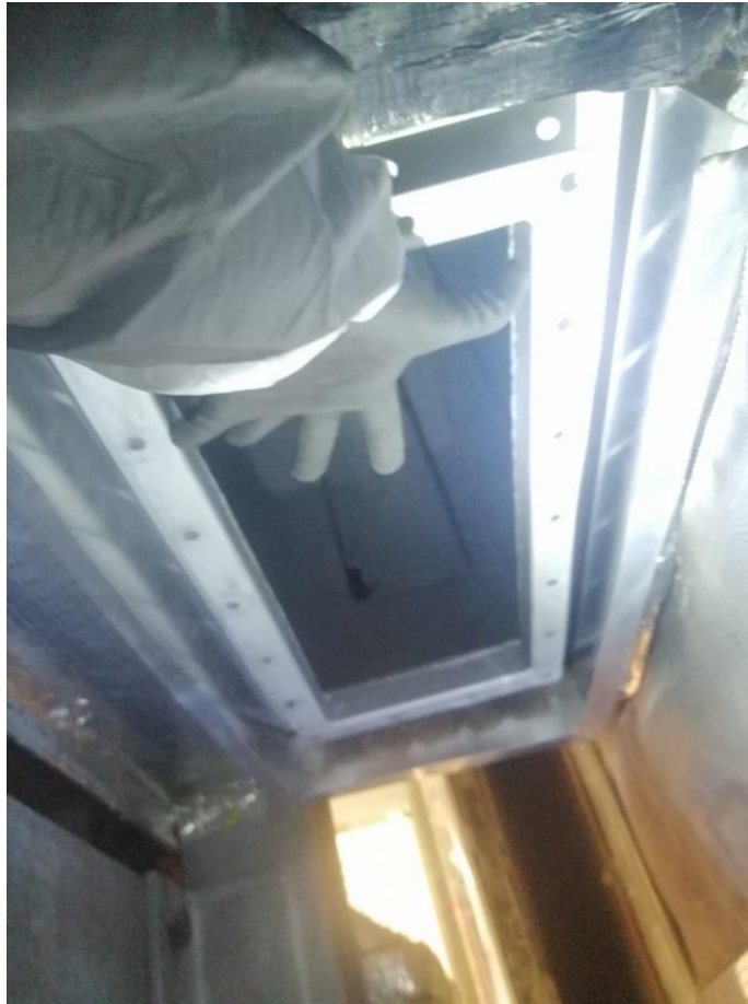
Photographs of an example of a fire damper accesible for visual inspection, but not for functional test
