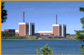
Olkiluoto power plant
