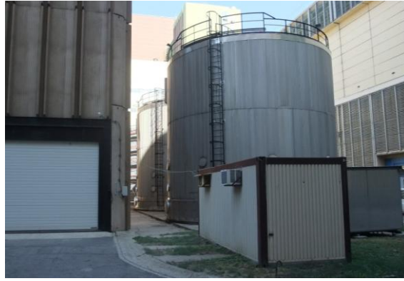
Figure 2-5: Demineralised water tanks of Installation II next to the wall of the service building
