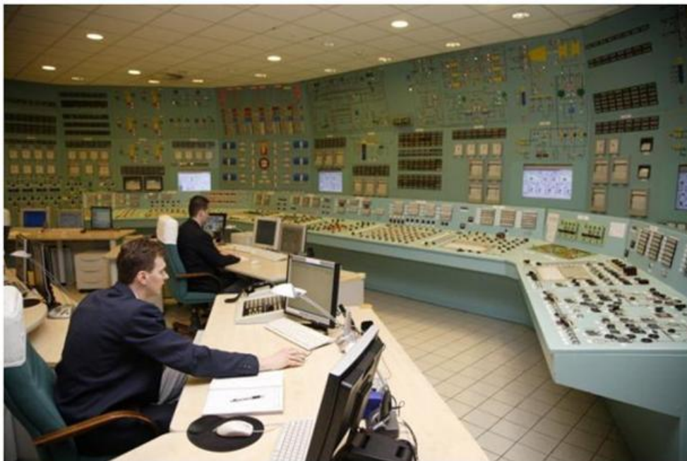
Figure 1-9: Picture of unit control room
