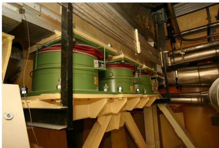
Figure 2-4: Reinforcement by viscous snubbers
