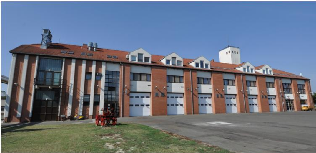
Figure 2-6: Fire brigade barrack on the NPP site
