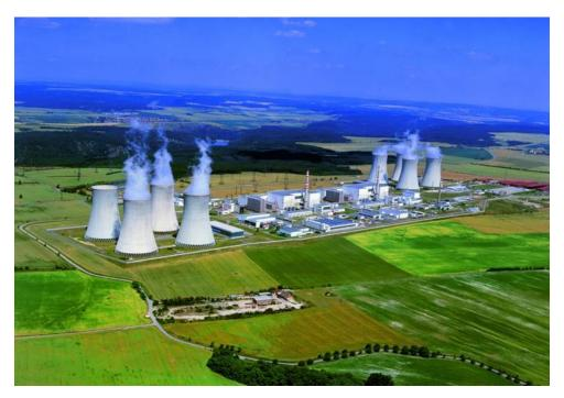
4 VVER 440 reactors (type V-213) with power 1 375MWt, resp. 1 444MWt The units were put into operation in the years 1985 to 1987
