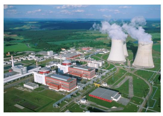
2 VVER 1000 reactors (type V-320) with power 3 000 MWt The units were put into operation in the years 2000 to 2002 Current Licenses issued in 2010/2012, valid till 2020/2022 Last PSR results reported in 2010
