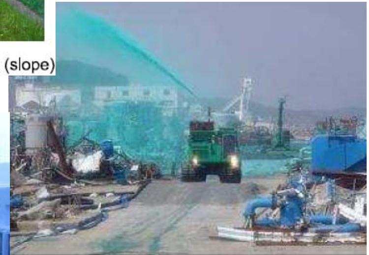
Dispersion of inhibitors around buildings of Units 1 to 4 by crawler dump
