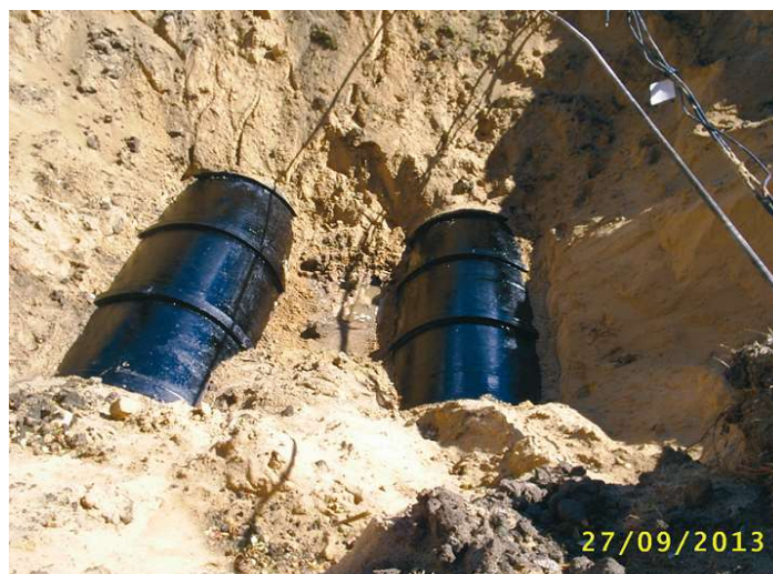
Figure 4.3 ESWS piping (visualization after excavation)
