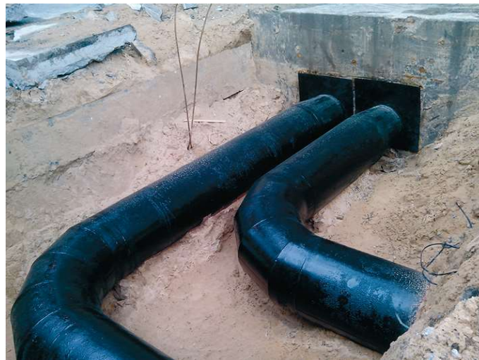
Figure 4.2 ESWS piping near well
