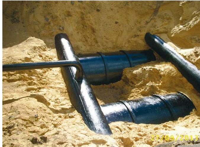
Figure 4.1 ESWS piping
