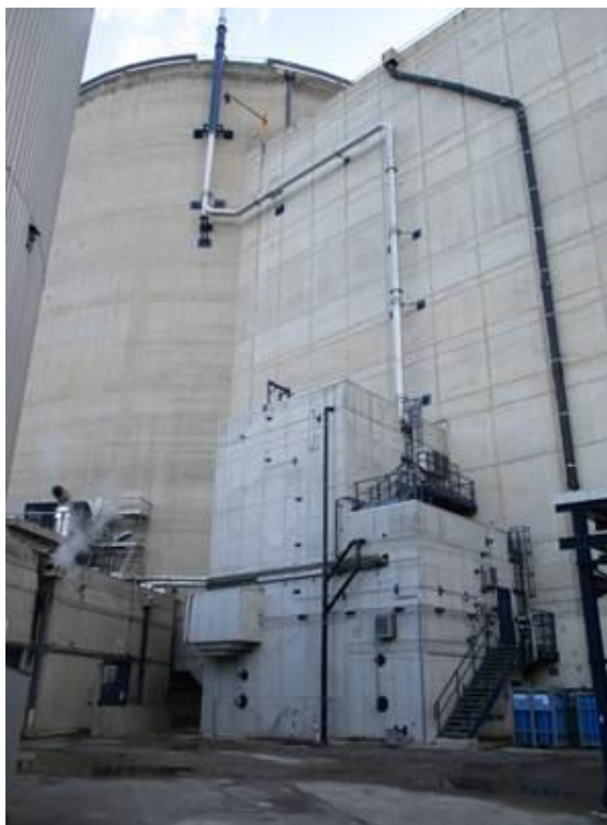
Figure 7 : Filtered containment venting systems of Tihange 3
