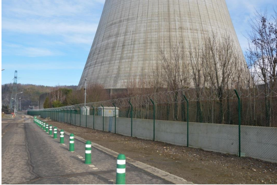
Figure 3: Peripheral protection of the site of Tihange against beyond-design flooding realized in 2015
