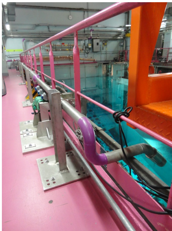
Figure 7: Alternative water supply installed in the Tihange 1 spent fuel pool in 2016.
