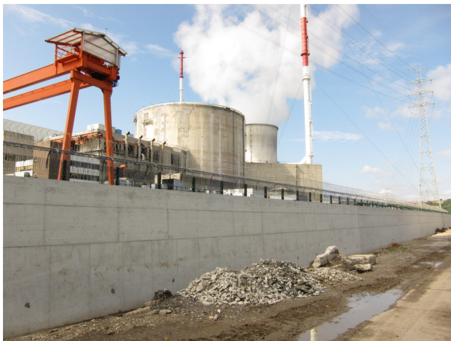
Figure 2 : Peripheral protection of the site of Tihange against beyond-design flooding realized in 2015
