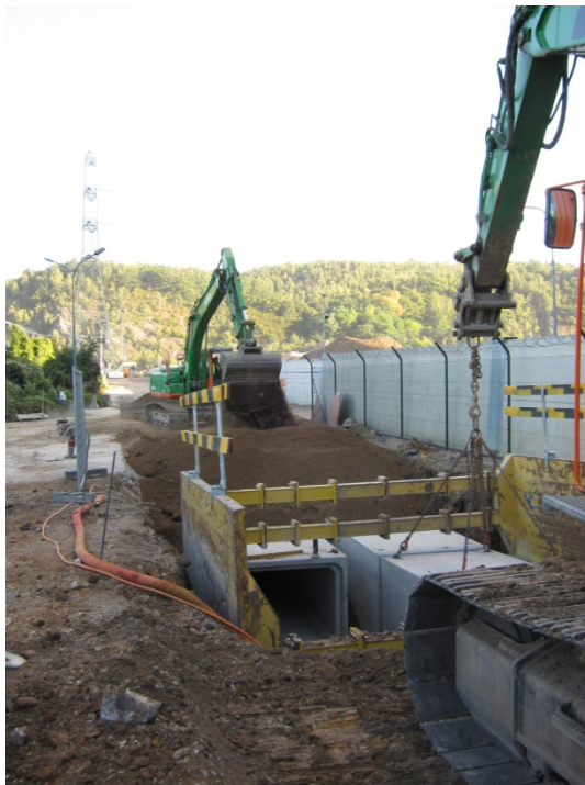
Figure 5 : Deviation of the underground municipal sewers
