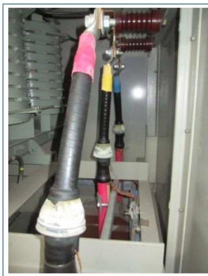
Figure 3A-6: Example of a termination arrangement (connection) at the Tihange NPP
