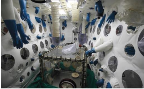
Glove boxes dismantling
