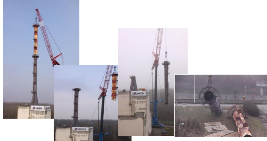
Caorso NPP Off-Gas dismantling
