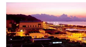
Ling Ao 2x990.3MWe 2x1080 MWe
